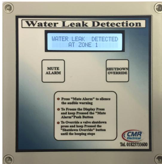
The LD4-2 range has been designed to monitor four independent zones in critical areas for water leaks via linier detection cables or spot sensors. Any number of spot sensors or a maximum of 50 metres of linier water detection cable can be connected to each zone.
