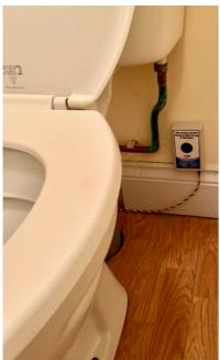
Between one and four remote sensors can be connected to an alarm unit, providing wire free water leak detection sensing in areas such as kitchen, bathroom, shower room basement or areas that running cables too would be difficult such as garages and out buildings. Providing no more than four sensors are installed, additional sensors can be added at anytime.
